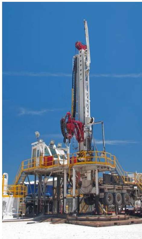
Figure 1: Lucas Soilmech 100 drill rig to be used at Cow Lagoon #1 well
